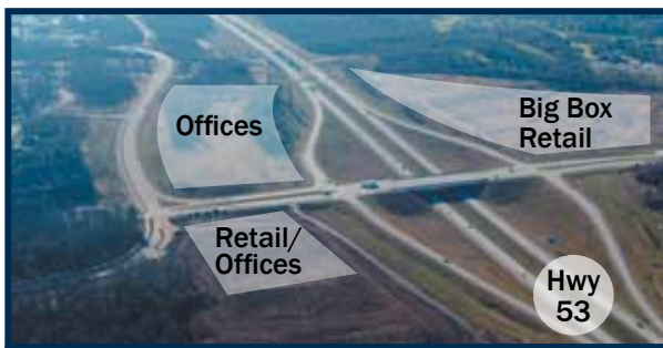
Aerial view of River Prairie Project and plans for the area.
